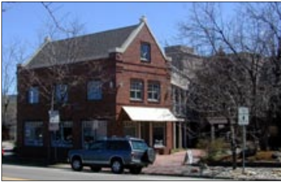
Mixed use commercial building with plaza
