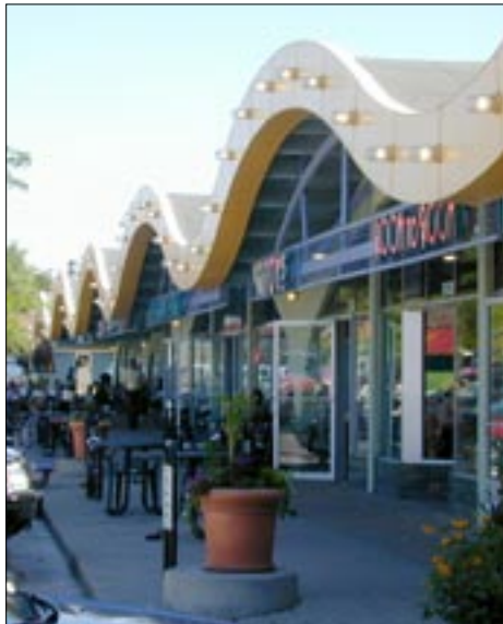
Rehabilitated commercial corridor storefront
