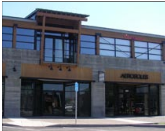
Mixed use commercial building
